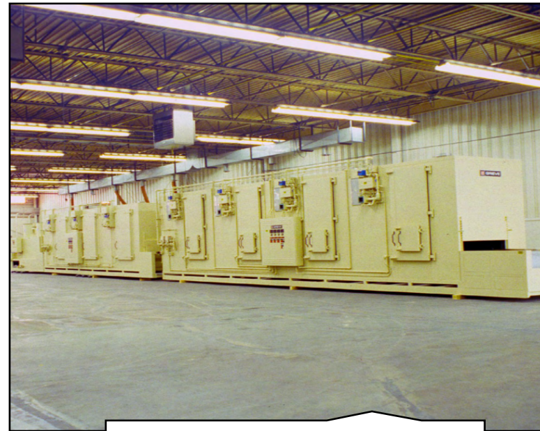
919 Custom Belt Conveyor Zones Door Modification
